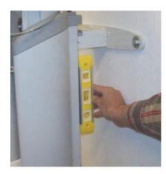
**8.** Mount the Vantage panoramic device to the floor: Select 2 cement anchors, 2 washers, and 2 nuts from the hardware kit. For wood floors, select 2 lag bolts and 2 washers. Drill through 1 hole in the floor base of the Vantage panoramic device using a 9.5 mm (3/8 in.) masonry bit. For wood floors, use a 6.3 mm (1/4 in.) bit.
